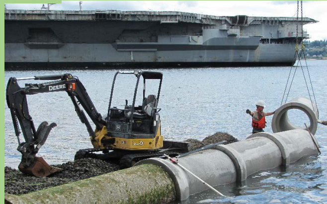
Stormwater outfall extension at Bremerton, WA
